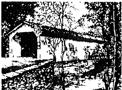
Green Sergeant's Bridge
