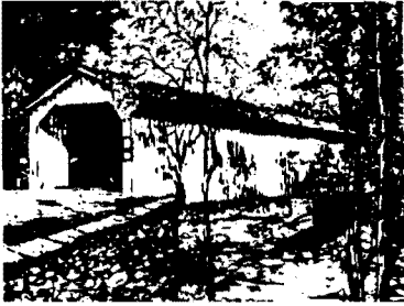
Green Sergeant's Bridge New Jersey's Only Remaining Covered Bridge
