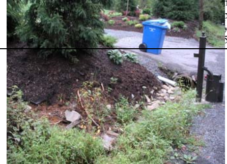
Lot drainage directed to swale.
