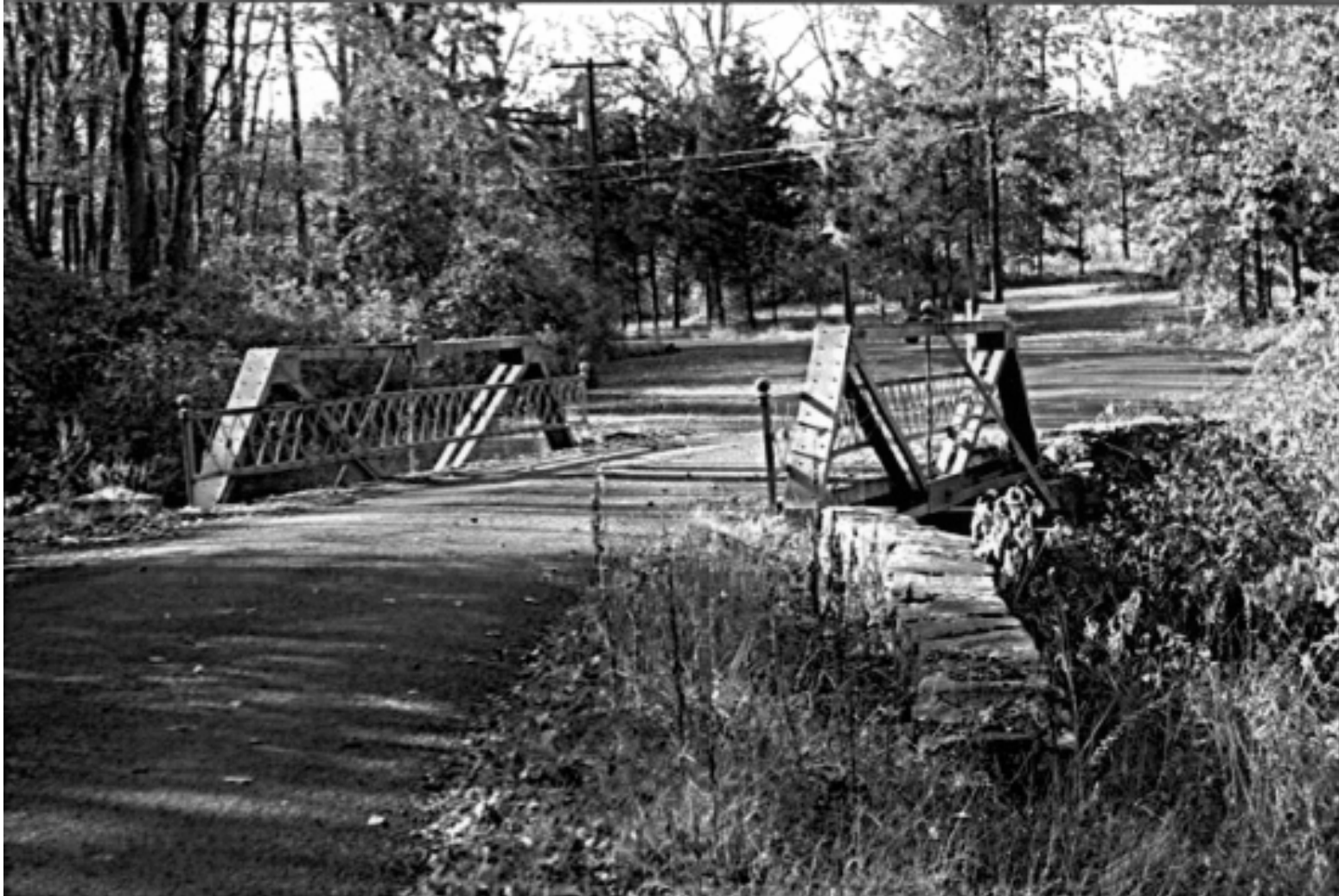
Metal Truss Bridge Example Delaware Township Historic Bridges MPDF Delaware Township, Hunterdon County, New Jersey
