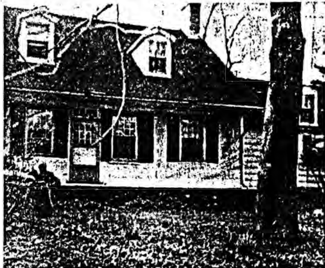
THIS REAR VIEW of the historic Van Wickle house on the Bogan property on Easton Avenue shows the 250-year-old house as it faces the Delaware and Raritan Canal. A footbridge across the canal to the towpath is one of the suggestions for improving the property should it be acquired and restored by the township as the Franklin Woman's Club is hoping.
